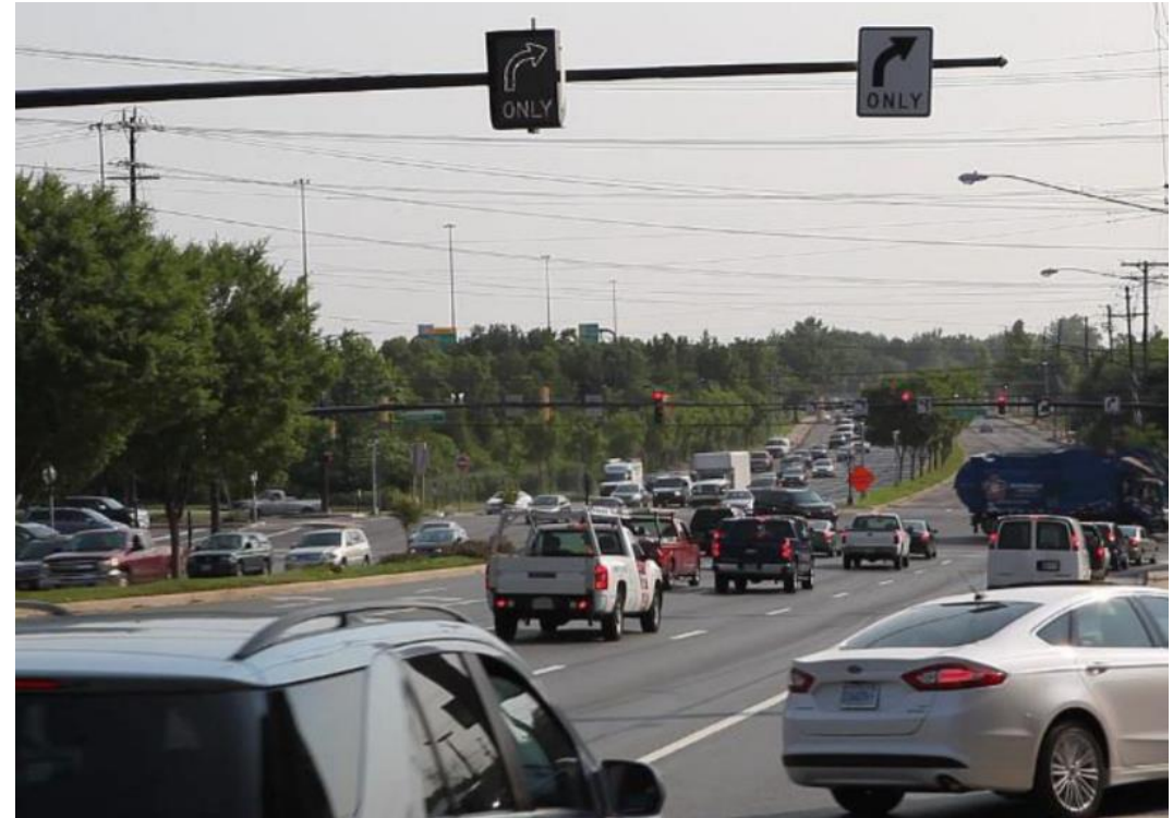
Exhibit 37-7 Upstream DLG Signage in Maryland
